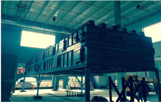
Installation of one of the belt dryers at WWRWRF
