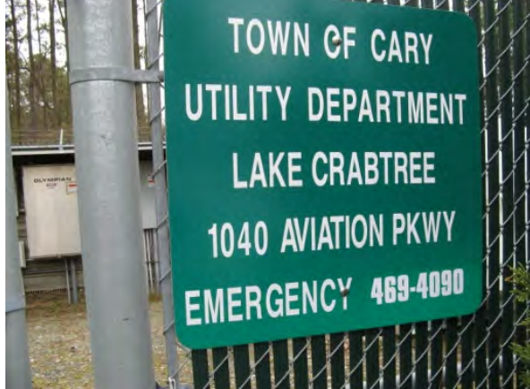
Lake Crabtree Pump Station
