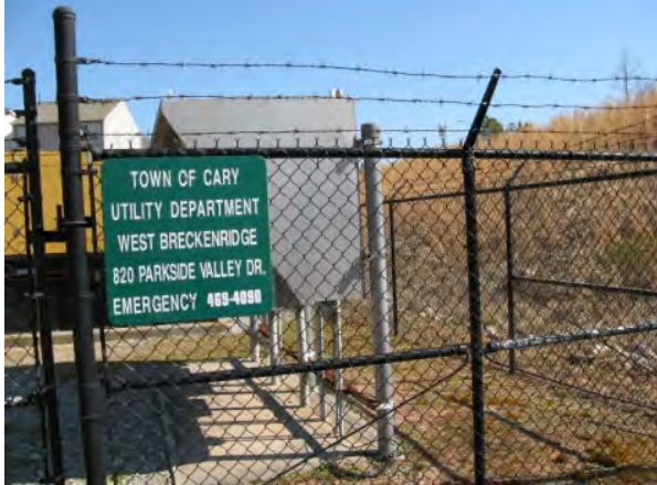
West Breckenridge Pump Station
