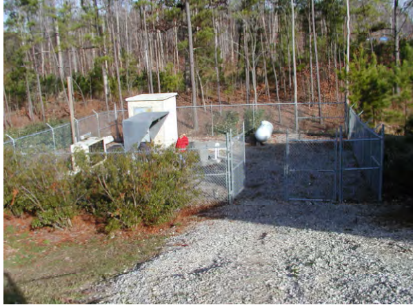
Westwood Park Pump Station
