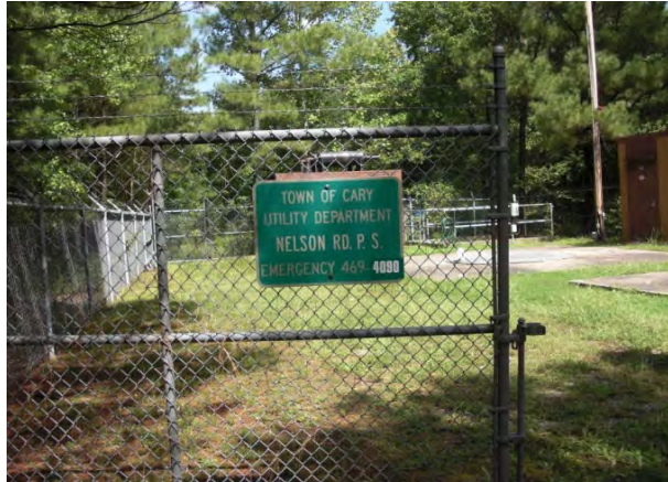
Nelson Road Pump Station
