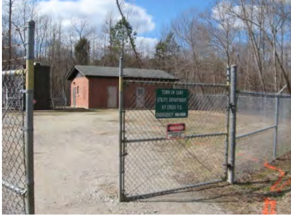
Kit Creek Pump Station
