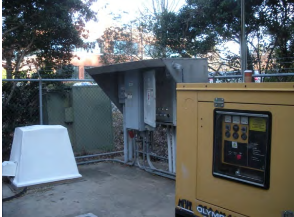
Jones Franklin Pump Station
