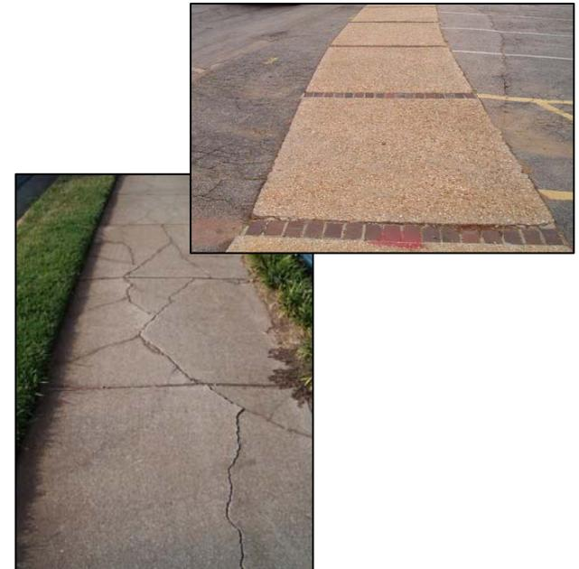
**Image 5-1.** Examples of various types of sidewalk material used in Cary. The top image is a combination brick and gravel decorative paver used in downtown. The bottom image is the more typical concrete sidewalk used elsewhere in Cary. Other materials besides concrete, such as rubber and asphalt, can be used to reduce the likelihood of cracking.
