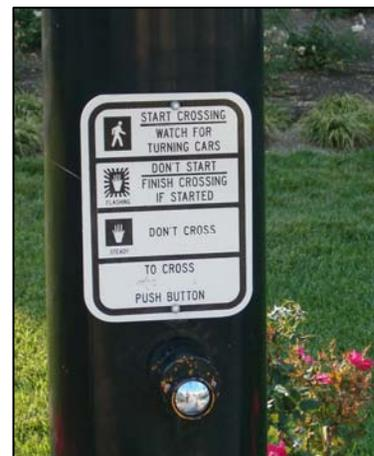
Image 5-3. Top image: An example pedestrian-activated signalized mid-block crossing. Bottom image: A guide for pedestrians to understand the meaning of the push-button signals.
