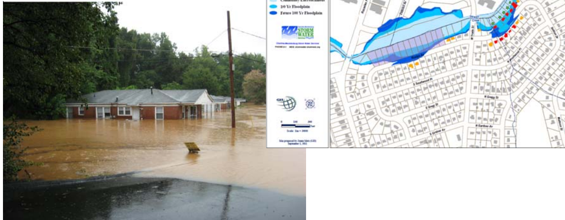
Figure 6.24 Flooded Building after August 2011 Event and Example Qualifying Criteria Map for Mecklenburg County Quick-Buy
