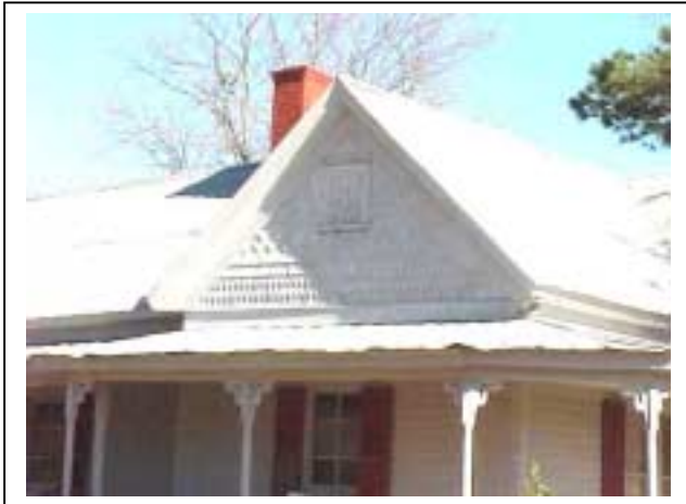
Gable detail on the Barbee-Williams House. Note decorative shingles and turned porch posts with sawn brackets.
