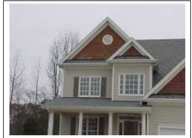
Gable detail on a home in Carpenter Village PUD. Note sash-over-sash windows, as in Barbee-Williams house.
