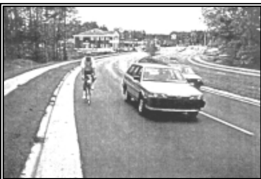
Wide Outside Lane along High House Road
